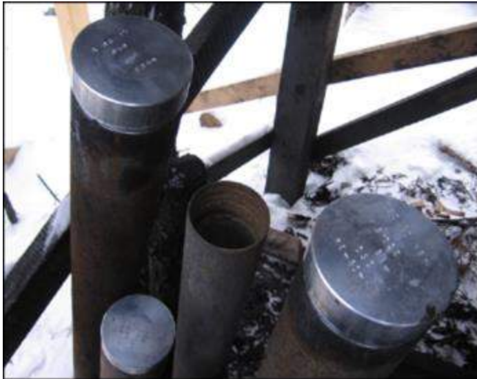
Figure 10-18: Capped Casing
